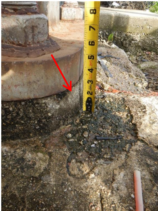
Figure 18. Grout installed under base plate of East Middle Pole.
