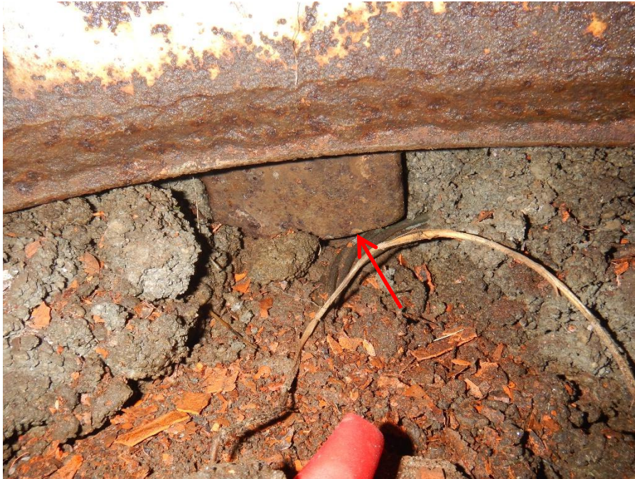
Figure 19. Leveling nut under base plate as seen through hand hole opening.
