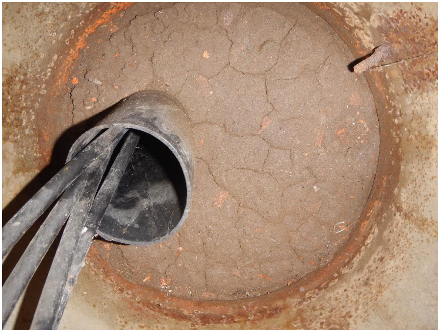
Figure 14. Soil inside pole as seen through hand hole opening.
