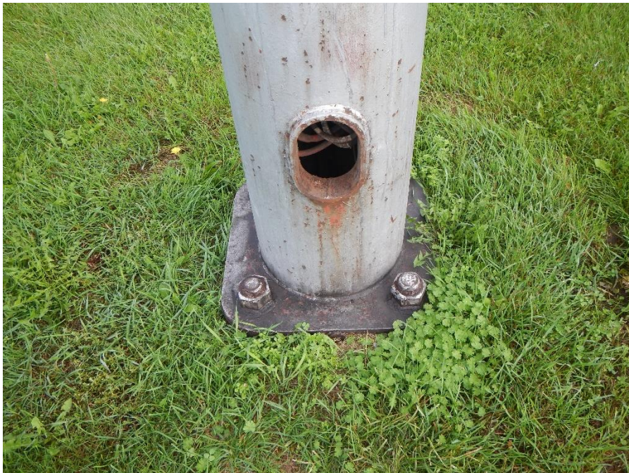
Figure 5. Typical hand hole at the base of a pole after removal of the cover. Note soil covering the top of the concrete foundation.
