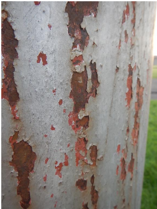
Figure 16. Uniform corrosion of pole at area of failed coating.
