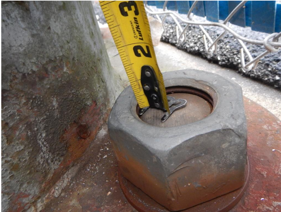
Figure 7. Partially threaded nut at West Middle Pole.
