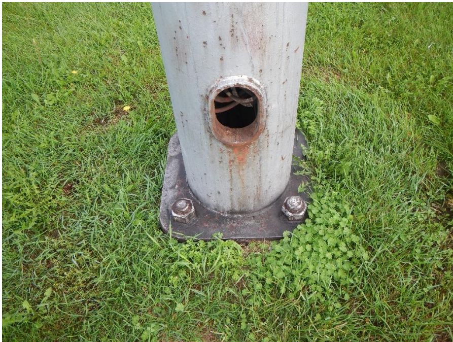
Figure 12. Soil covering foundation and grout at Northwest Pole.
