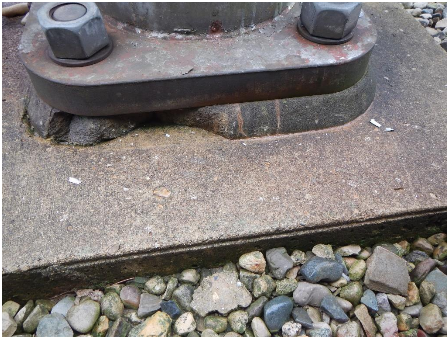
Figure 20. Spalled grout under West Middle Pole.
