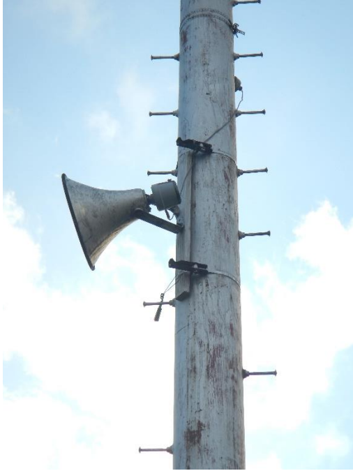
Figure 21. Speaker attached to Southwest Pole via wood blocking and steel straps.
