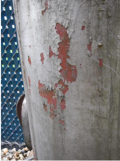
Figure 15. Failed coating on exterior surface of pole.
