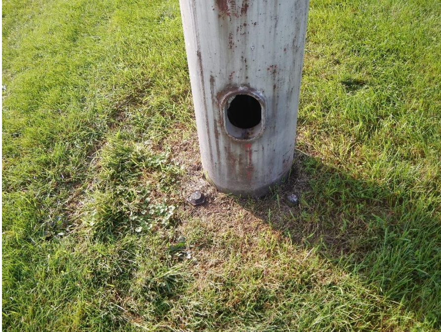
Figure 11. Soil covering base plates and part of anchor bolts and nuts.
