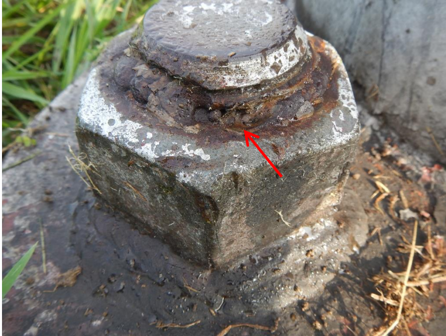
Figure 9. Section loss of anchor bolt at weld installed between nut and anchor bolt.
