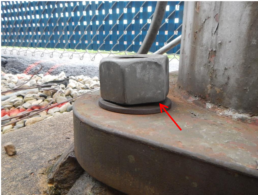
Figure 6. Nut at West Middle Pole with a gap between the nut and washer.
