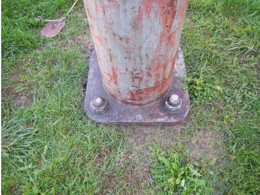
Figure 4. Base plate and anchor bolts at base of pole.
