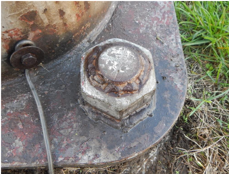
Figure 8. Nut welded to anchor bolt and base plate.
