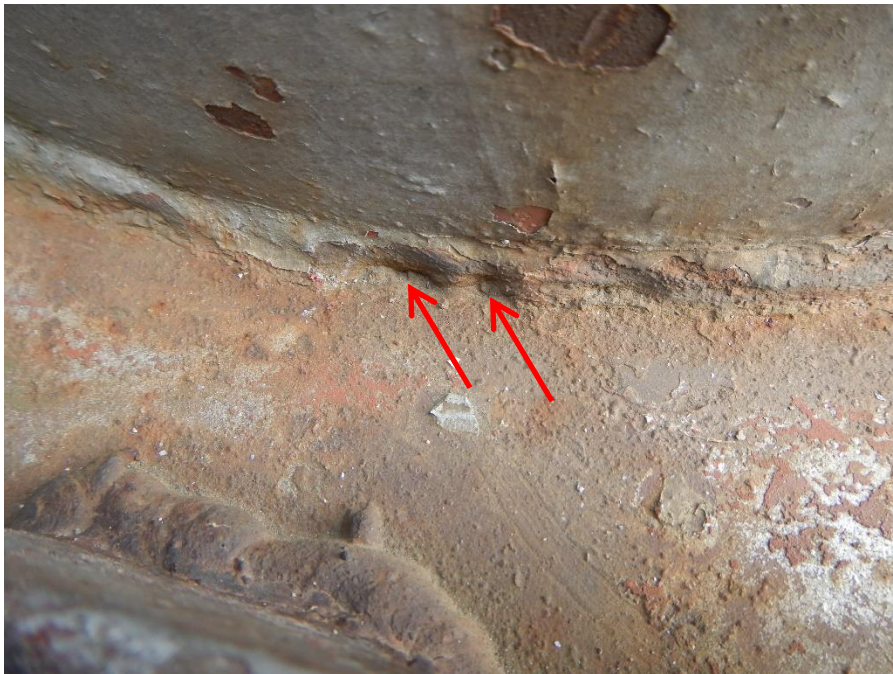
Figure 10. Undercut and poor profile at weld between pole and base plate.
